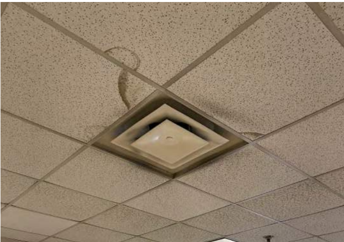
FIGURE 3: Acoustic ceilings show some signs of water damage from concealed piping. Dust marks adjacent to diffuser suggest duct cleaning is required.
