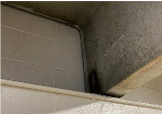
FIGURE 3: Precast concrete has the most integrity in protected areas; within open areas of the garage there is visible damage from equipment hitting the bottoms of the beams.
