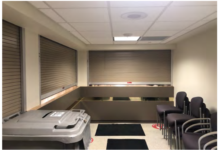
FIGURE 2: Service counters are hidden and feature dated, less durable finishes. Counter heights do not have portions that comply with accessibility requirements for lower service areas.
