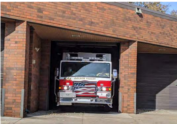
FIGURE 11: Apparatus bay doors are undersized for modern equipment, leading to difficult entry and exits during a call.
