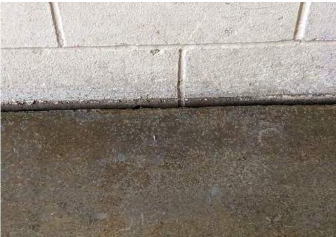
Figure 15: Some signs of separation and settling appear along the exterior walls of the apparatus bay. Dimension of settlement is not concerning at this time.
