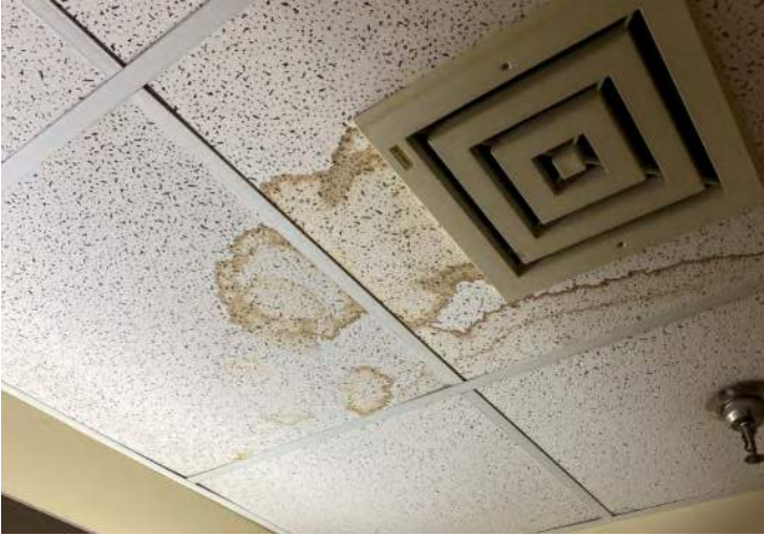
FIGURE 7: Acoustic ceiling tiles in the locker rooms and offices show signs of water damage from concealed piping above.
