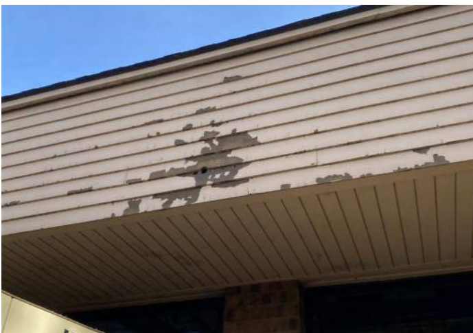
FIGURE 5: Wear and damage from birds is common in the exterior fascia.
