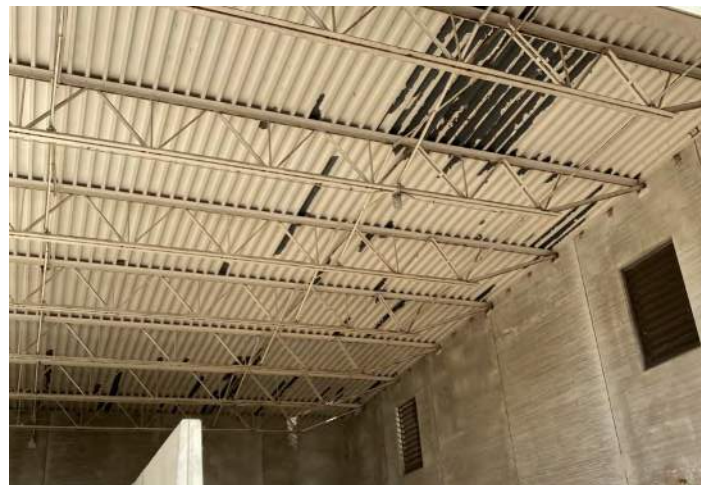
FIGURE 4: The salt and sand storage structure shows some wear on the metal decking at the roof.
