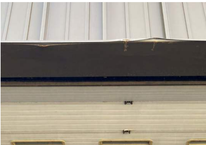
FIGURE 5: Some damage from equipment appears above the garage doors in the metal cladding.
