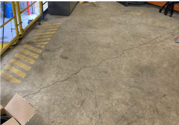
FIGURE 5: Some cracking also appears in the second floor slab.
