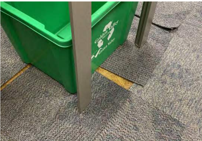
FIGURE 11: Carpet tile in the Police Dept record storage/work room is loose, with no permanent adhesion.
