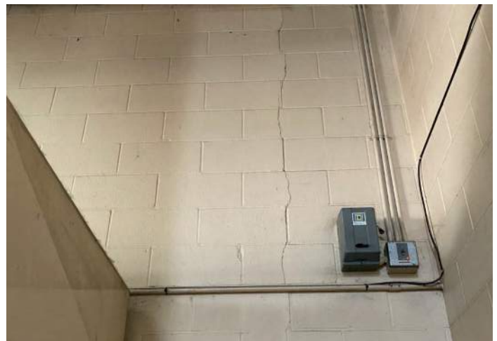
FIGURE 4: Cracking also appears on the masonry wall separating the Parks garage from the Police auxiliary garage.
