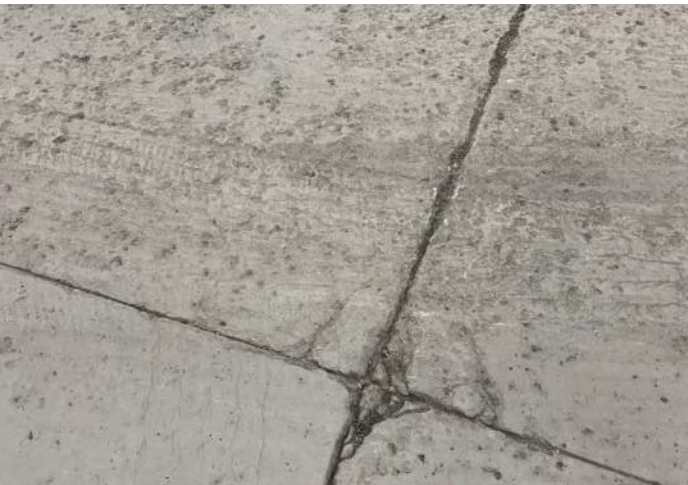
FIGURE 9: Visible damage and wear on the floors is common throughout the Streets department garage.
