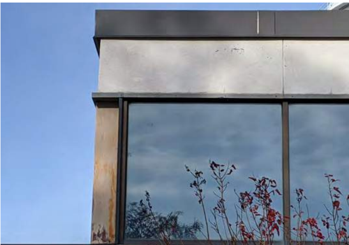
FIGURE 11: Some signs of metal oxidation and staining on the exterior.
