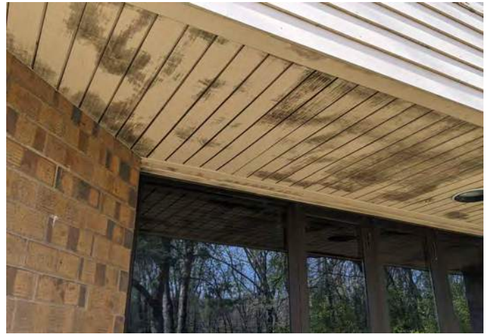
FIGURE 2: Signs of wear and moisture are visible at exterior wood soffits and fascia.
