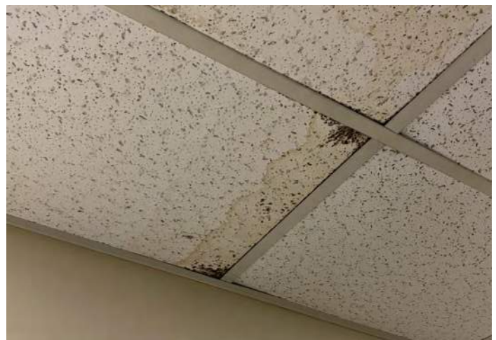
FIGURE 6: Acoustic ceiling tiles in the locker rooms and offices show signs of water damage from concealed piping above.
