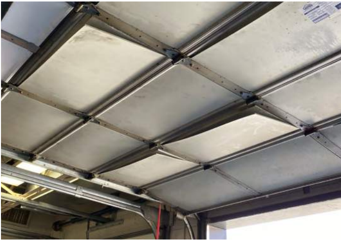
FIGURE 13: Insulated panels on the Police Department garage doors are delaminating.
