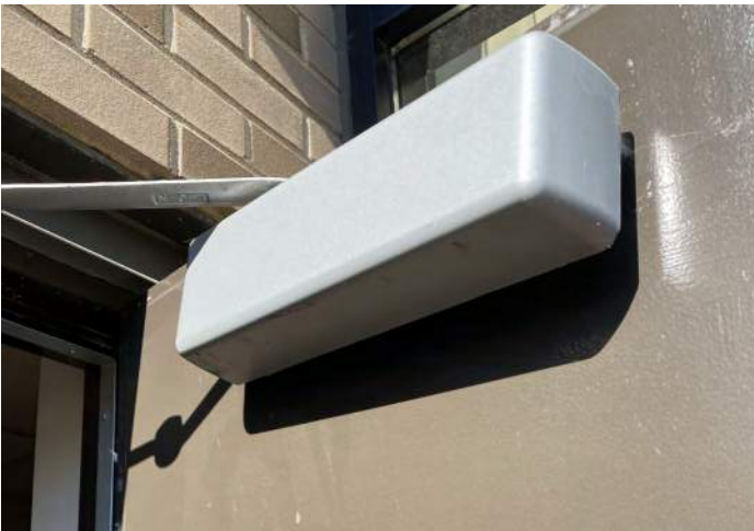
FIGURE 9: Overhead door closer on an exterior door is loose at this heavily-used access point.
