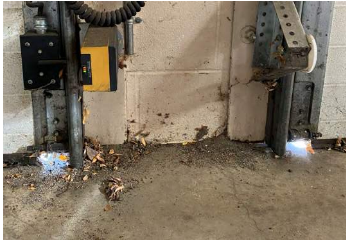
FIGURE 14: The seals on the Police Department garage doors have worn and now allow outside air in.
