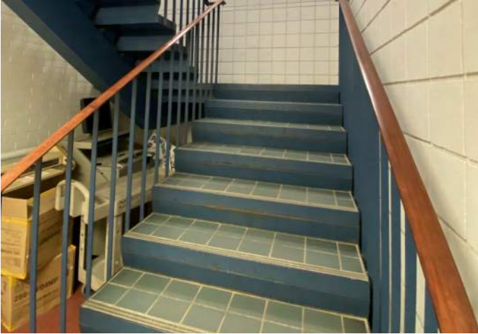
FIGURE 7: Finishes on the floor tile in the stairwell are visibly worn. Guardrails and handrails are non-compliant in detail with ADA.
