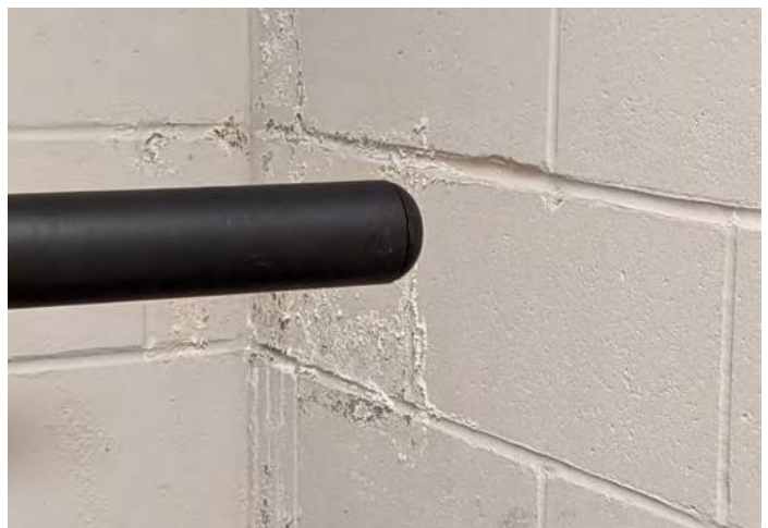
FIGURE 18: Interior walls at the basement level show some signs of moisture damage and efflorescence.
