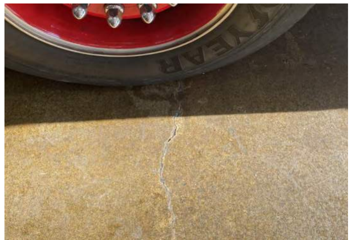
FIGURE 6: Some visible cracking appears in the apparatus bay floors.
