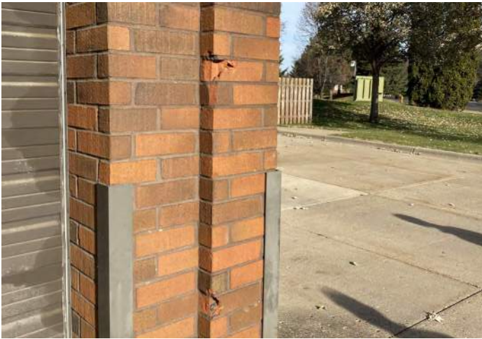
FIGURE 1: Exterior brick finish shows some signs of accidental damage from vehicles leaving and entering the apparatus bay.
