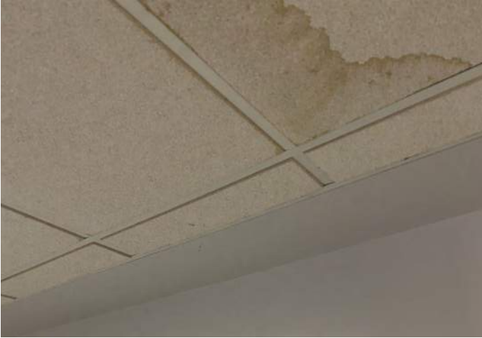
FIGURE 7: Some signs of water damage are apparent in the ceiling systems. This indicates minor issues with HVAC piping above.
