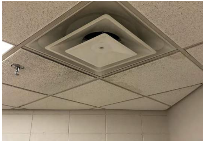
FIGURE 8: Signs of moisture and mold problems are present in the ceiling tiles.
