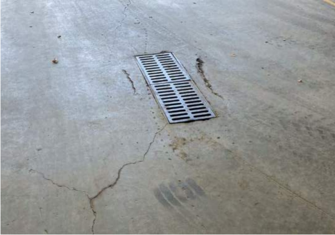
FIGURE 1: Some cracking is apparent at the trench drains.
