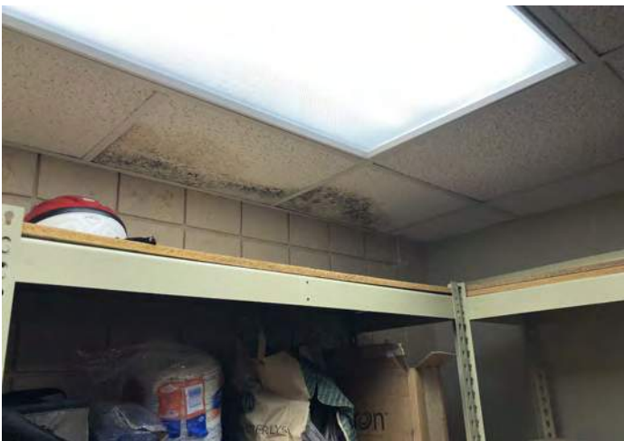
FIGURE 3: Some signs of water damage are present in limited areas in the lower level ceilings, indicating issues with piping above ceiling.
