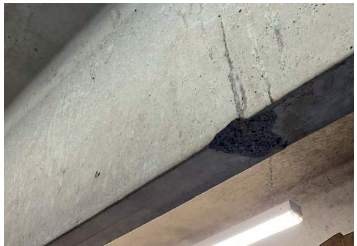
FIGURE 4: Damage to the bottom of a structural beam within the open garage area from the equipment adjustments necessary to nestle and park vehicles and equipment.
