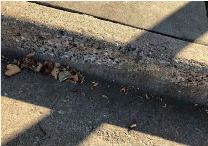
FIGURE 1: Some damage from equipment is visible on the curbs throughout vehicle driveways and parking areas shared with City Hall, Police, and Fire.
