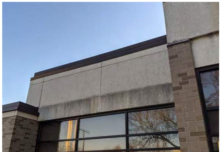
FIGURE 16: West-facing EIFS shows some signs of age at a superficial level.
