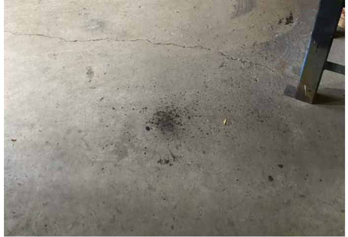
FIGURE 2: Cracking and other wear is visible throughout the garage floor.
