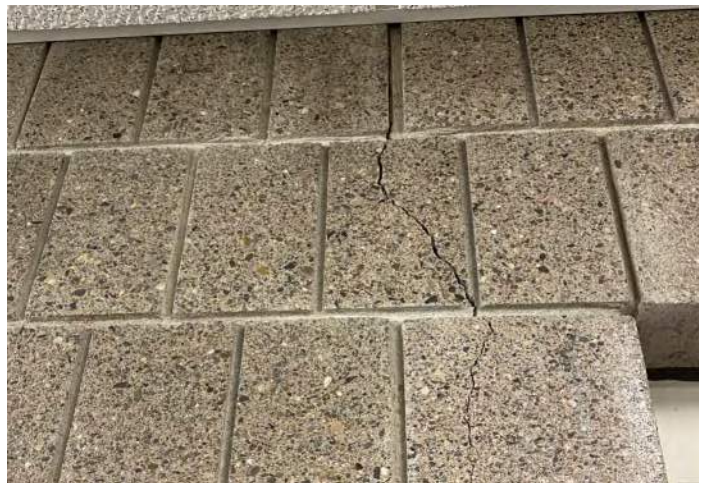
FIGURE 12: Some visible cracking appears in the dayroom walls.
