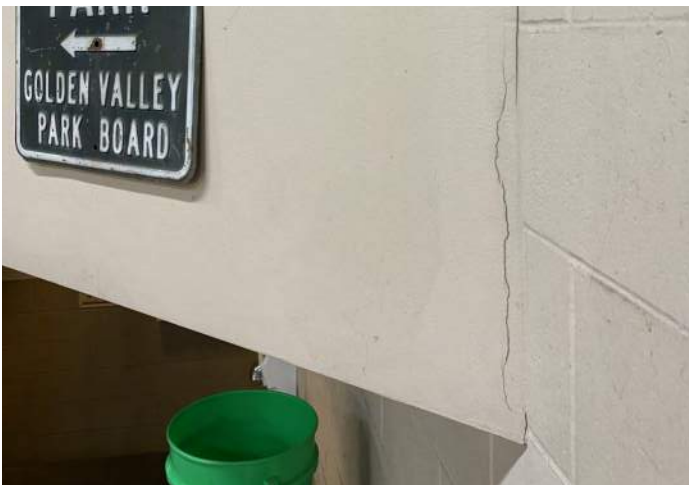
FIGURE 3: Some visible cracking appears on the interior walls in the Parks department garage.
