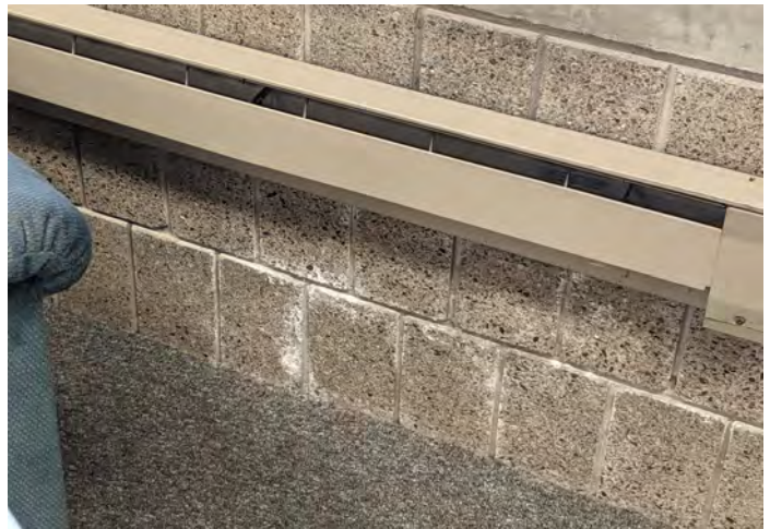
Figure 16: CMU walls in the dayroom show signs of efflorescence.
