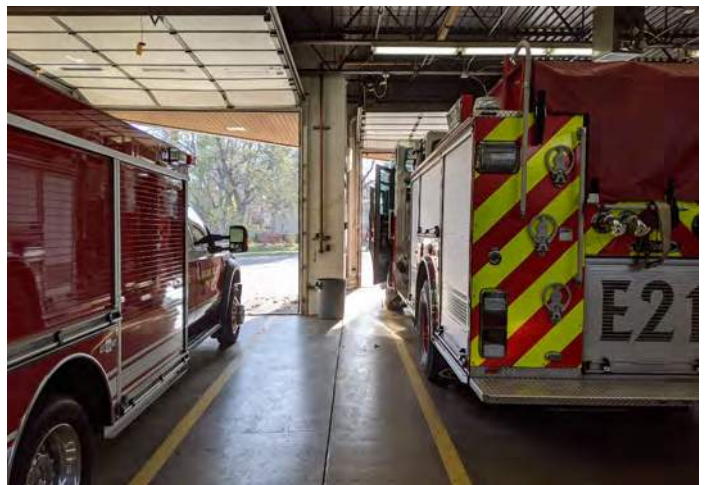
FIGURE 4: Staggered layout of the apparatus bay, along with narrow bay doors, leaves little room for vehicle doors to open, or for adequate turn-down space.
